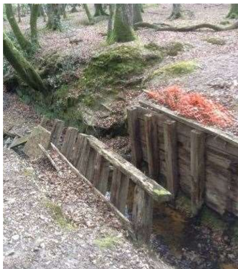
Figure 5.3: Collapsed pedestrian bridge (SU 22602 15796)
